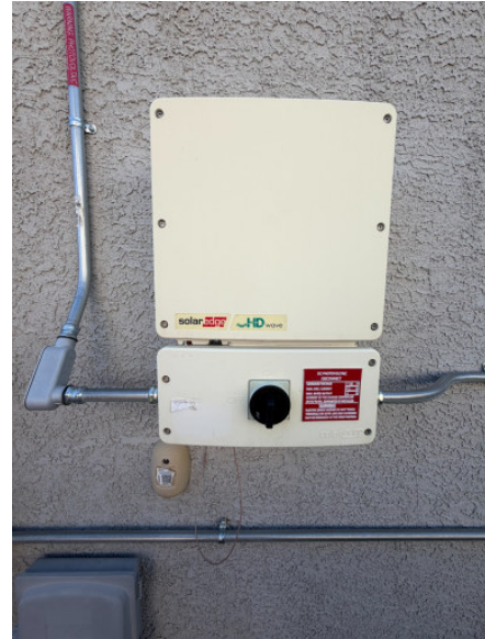
SOLAREEDGE INVERTER
